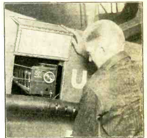
Mr. F. E. Gray, radio engineer of the National Aircraft Transportation Company, inspecting a Stromberg-Carlson radio receiver installed in a mail plane.
